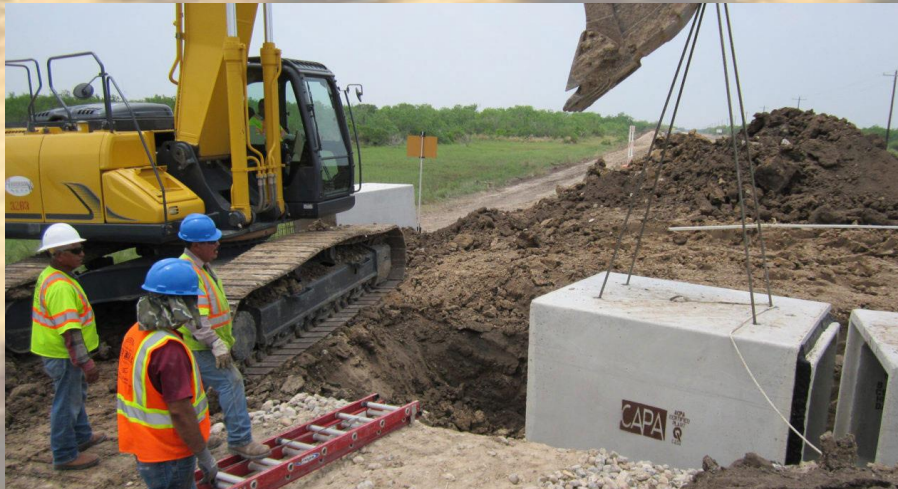
Construction on an ocelot wildlife crossing in Cameron County, Texas. Image: US Fish and Wildlife Service
